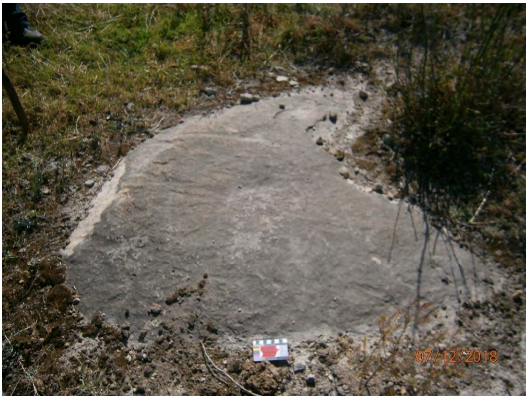
Figure 20: Machine damaged sandstone block rock in Stage One 7 December 2018
