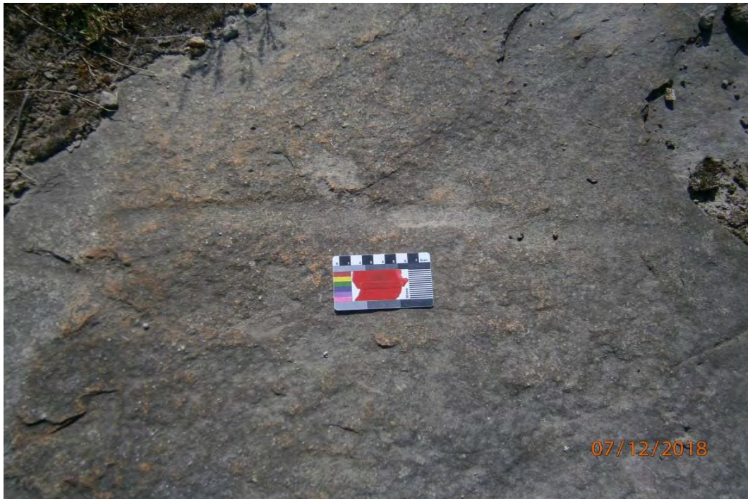
Figure 19: Machine damaged sandstone block in Stage One 7 December 2018
